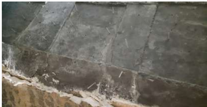
Cooler Bull Nose after Refractory Work
