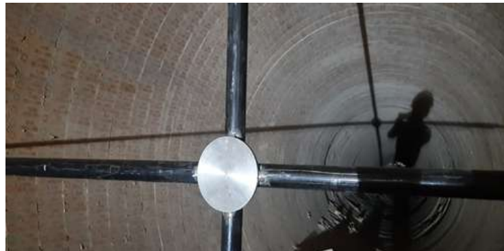
Bricks Lining Completed
