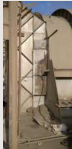
Kiln side wall patch work done
