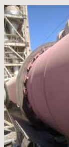
Kiln Outlet tyre shimming done
